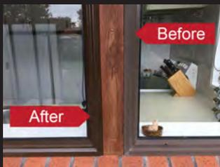
Anodized and powder-coated aluminium window frames, extrusions, garage doors, fencing and guttering can fade and oxidize from exposure to the sun. They can get ugly pits from salt corrosion if located near the ocean. When the finish is removed by harsh chemicals, stucco or mortar, it can have white stains which ruin the look of the anodized aluminium. There are many colours of anodized and powder coated aluminium which fade, chalk and look dull.
